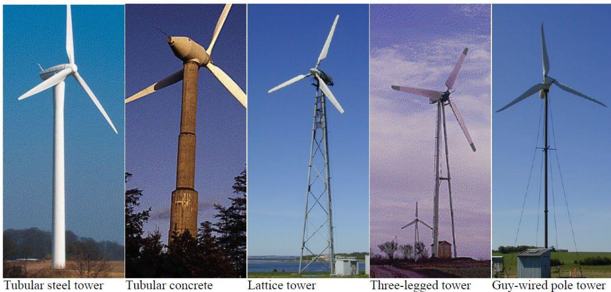
Figure 5. Commonly Used Turbine Structures
